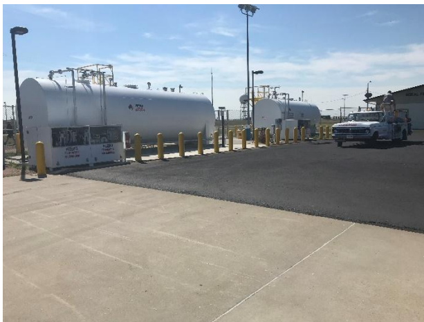
Figure 1-12. Jet A and 100LL ASTs
