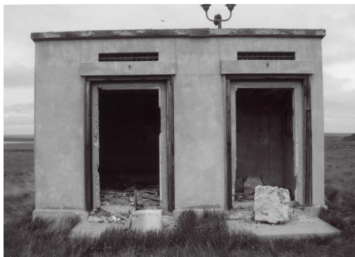
Figure 1-4. Glasgow Army Airfield Norden Bombsite Storage Vault.
