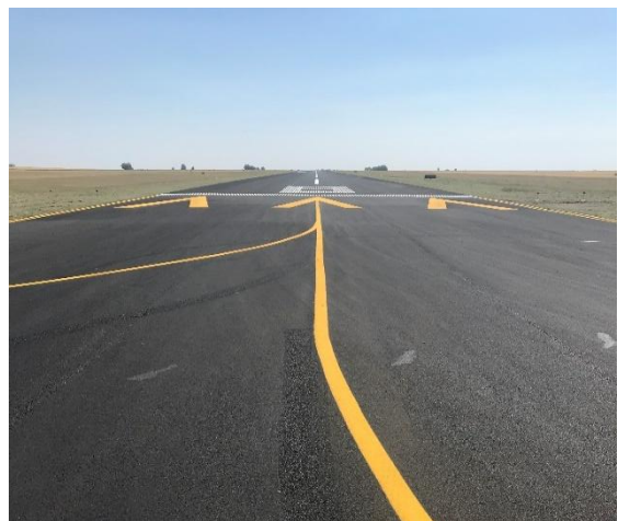
Figure 3-3. Lead-in taxiway to Runway 8
